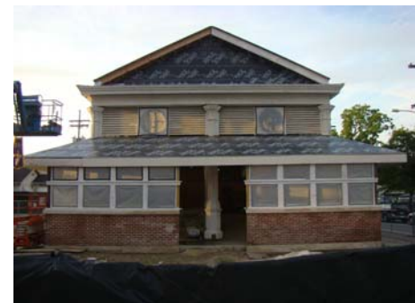
St. Roch Market: an exceptional renovation
